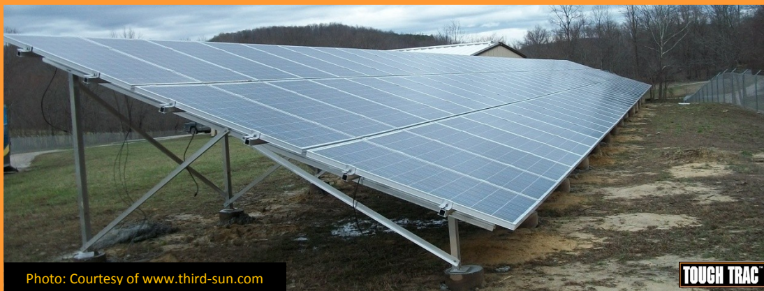
VERTICAL SUPPORT WITH WELDED BASE PLATE
